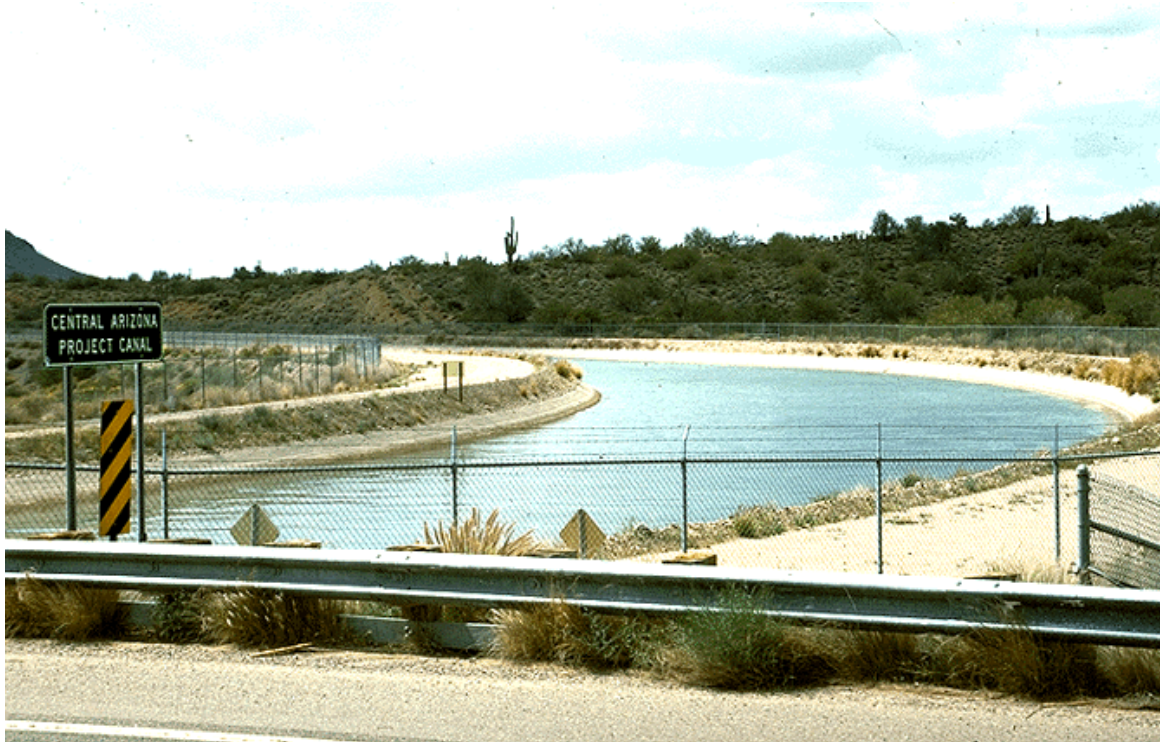
Figure 9. Central Arizona Project – 1.5 million acre feet per year. Provides water to 314,820 acres of irrigated agricultural land (a total of 127,000 hectares).
